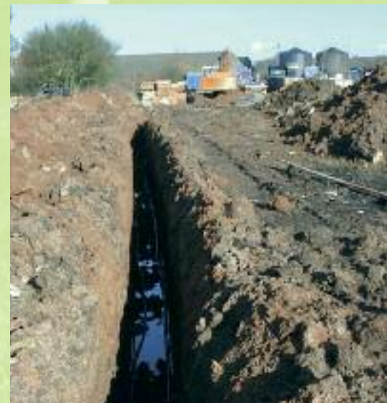
Work on a geothermal system.
